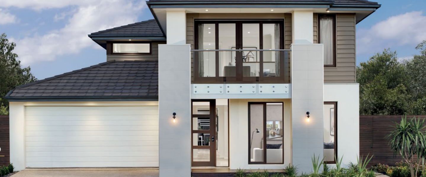
Lonsdale 44 Lincoln Façade Image courtesy of Henley Builders.
