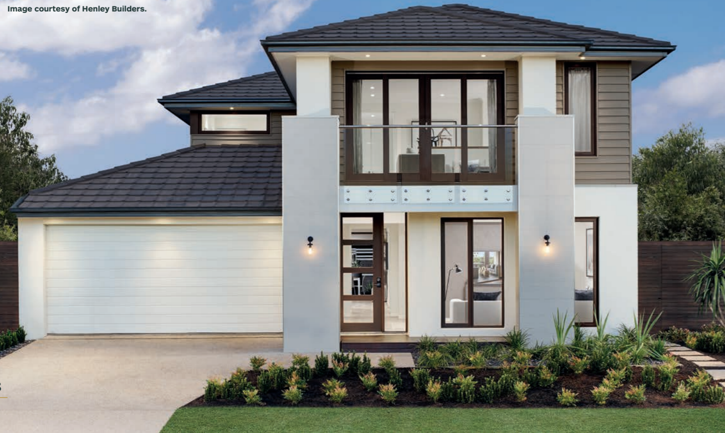
Lonsdale 44 Lincoln Facade Image courtesy of Henley Builders.
